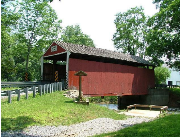
Rock Covered Bridge in Pennsylvania received $1.1 million in federal funds for renovations.
